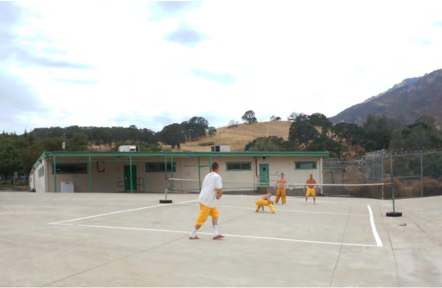
Figure 53: The dormitories are relatively open, but are not designed for full visual supervision. They are appropriate only as low-security housing.
