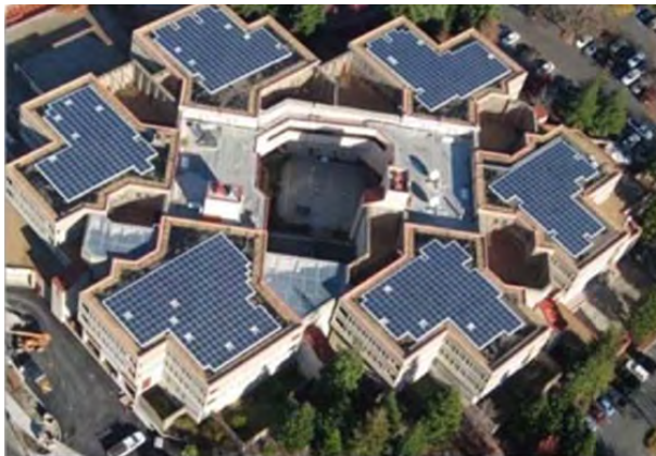
Figure 4: Aerial view of the MDF facility
