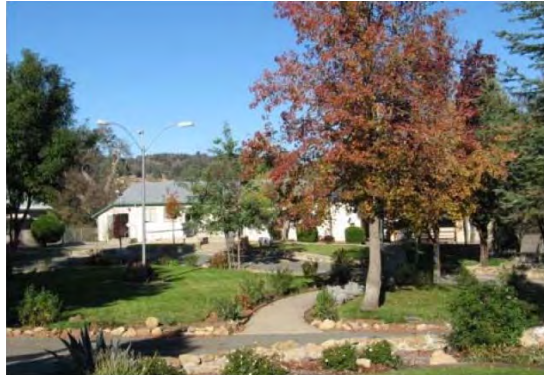
Figure 11: Exterior of MCDF Administration Building
