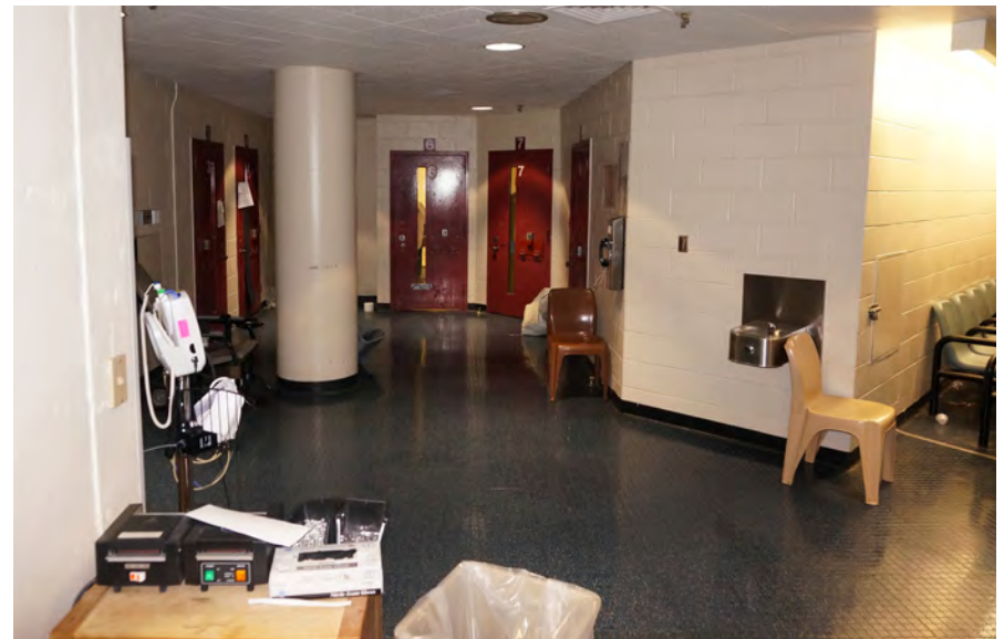
Figure 44: The complex angular layout of Reception & Release makes it impossible to supervise from one location.
