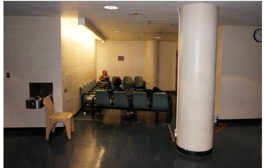
Figure 43: The view to the open seating area from the officers station in Reception & Release is partially obscured by a large structural column.
