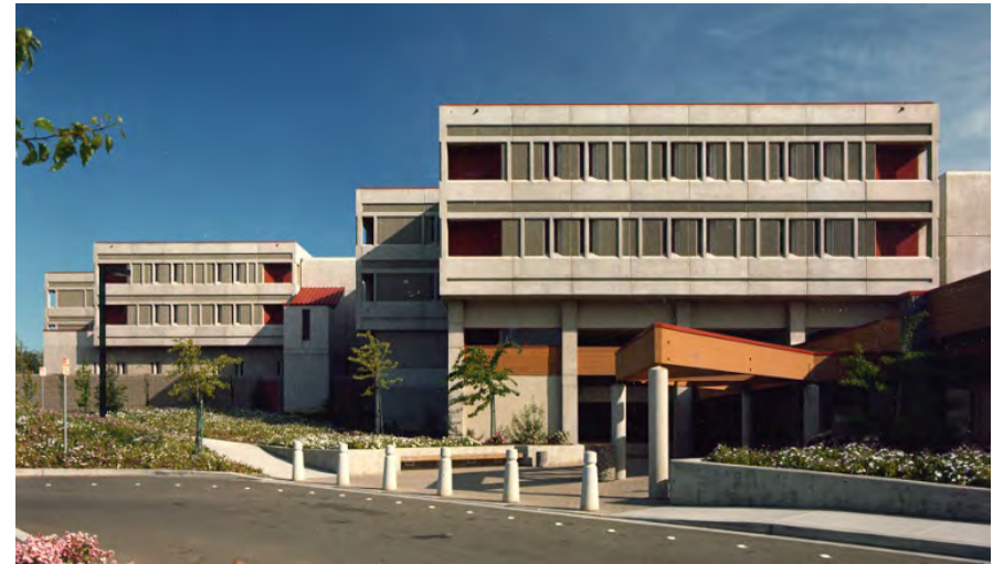
Figure 2: Exterior view taken shortly after construction completion
